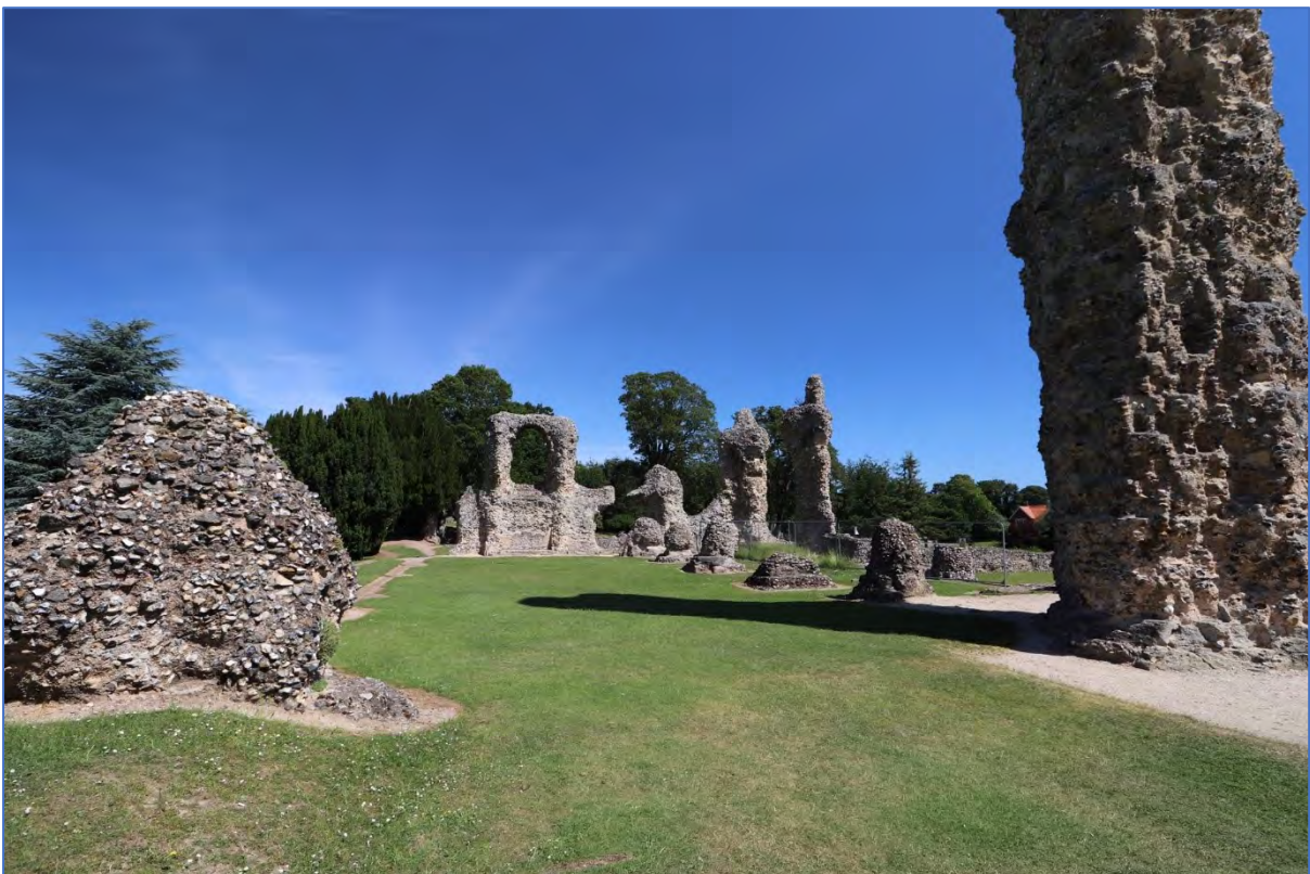
Figure 102: The north transept, looking north, showing the piers of the eastern aisle of the transept and the remnants of the cloistral buildings beyond.
