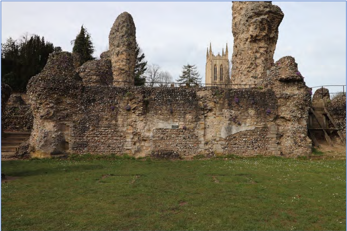
Figure 96: The western wall of the crypt, looking west, showing the wall scars of the former arcading and the locations of the northern and southern staircases into the crypt.
