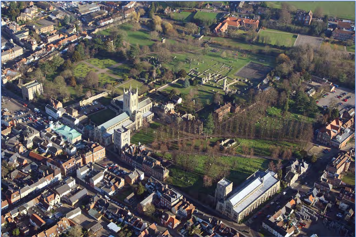
Figure 130: Aerial view of the Great Churchyard looking north-east, showing St Edmundsbury Cathedral, St Mary's church and the Chapel of the Charnel. (© Mike Page, reproduced with permission)
