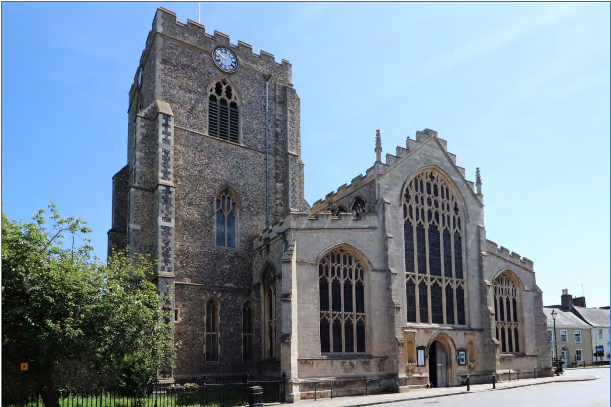
Figure 134: St Mary's church, looking westwards, showing the offset northern tower and the traces of the precinct wall extending to the north of the tower.
