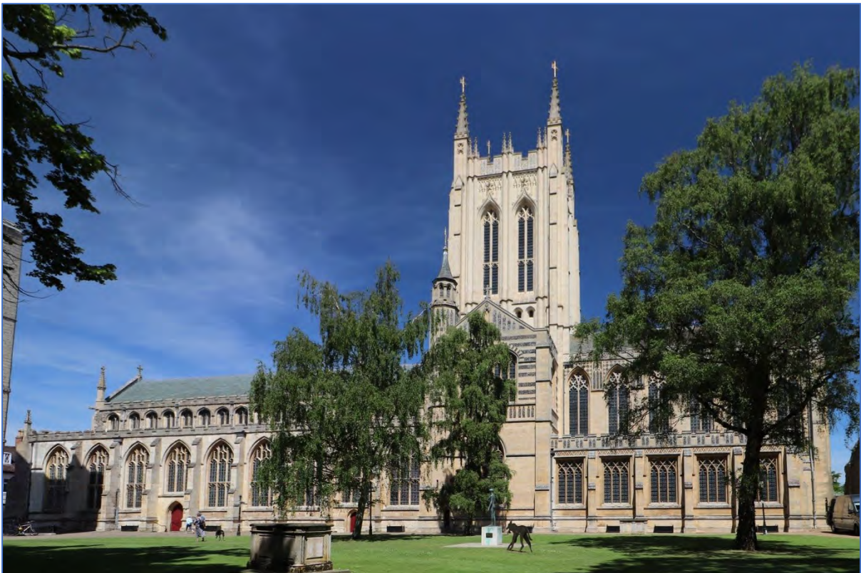
Figure 133: St Edmundsbury cathedral looking north-west. The area excavated by Radford and Dufty in the late 1950s lies under the nearest corner of the building.
