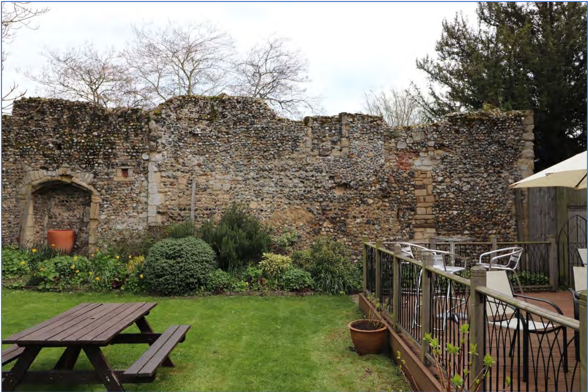
Figure 129: The eastern wall of the Cathedral Garth, looking east, showing the preserved gable end of a medieval building, with a blocked doorway to the north..
