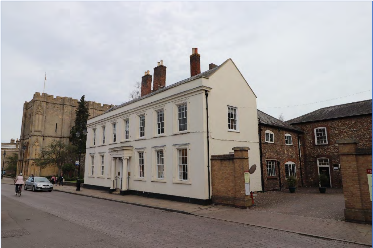
Figure 145: Abbey House looking north-east, with the Abbey Gate beyond and extensions to the rear.
